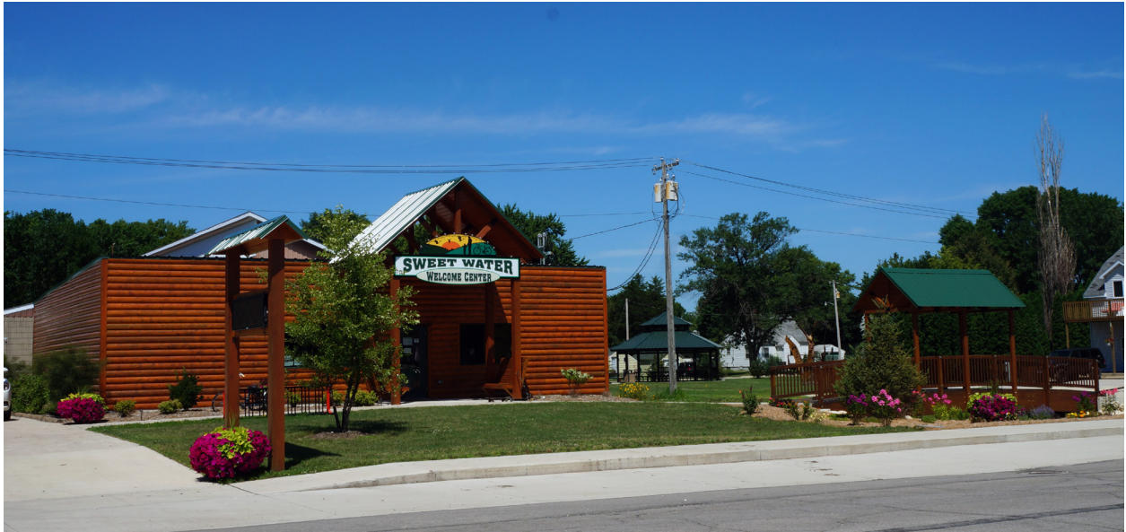
The Sweet Water Trail trailhead and welcome center was built completely by volunteers of all ages.
