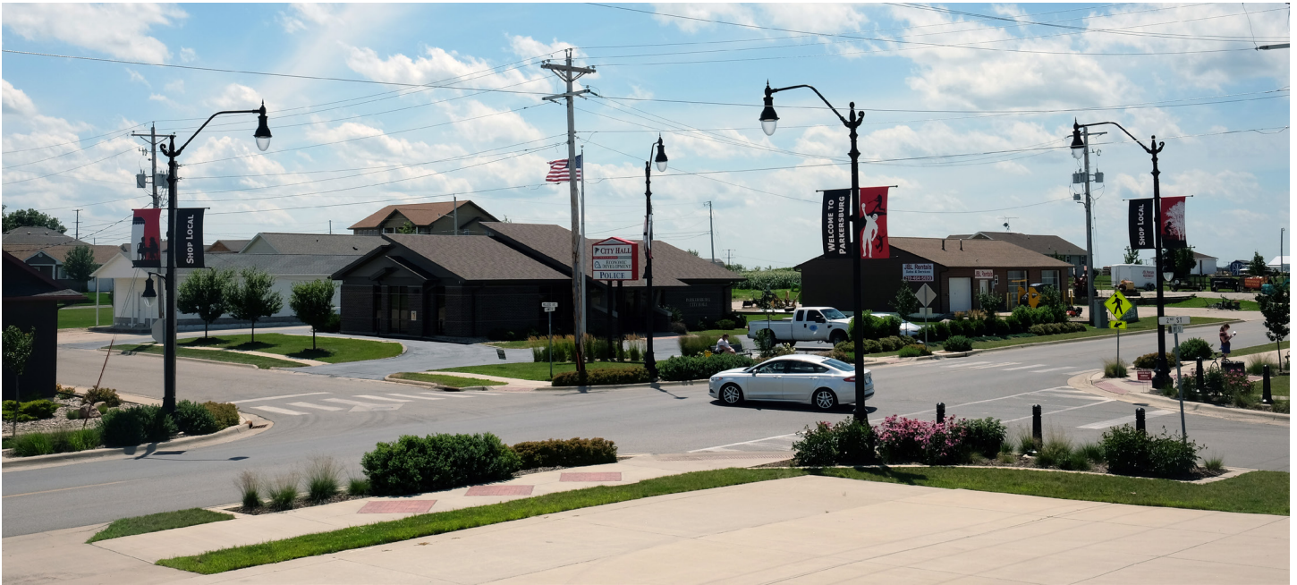
The landscape design for the Highway 14/57 corridor through Parkersburg includes curb ramps, crosswalks, pedestrian-scale lighting, and vegetation.
