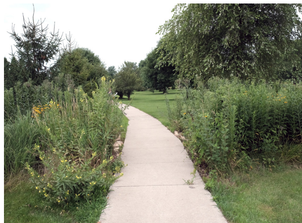
Volunteers lay cement for the trail in Box Park (top) before planting a bioswale (bottom).
